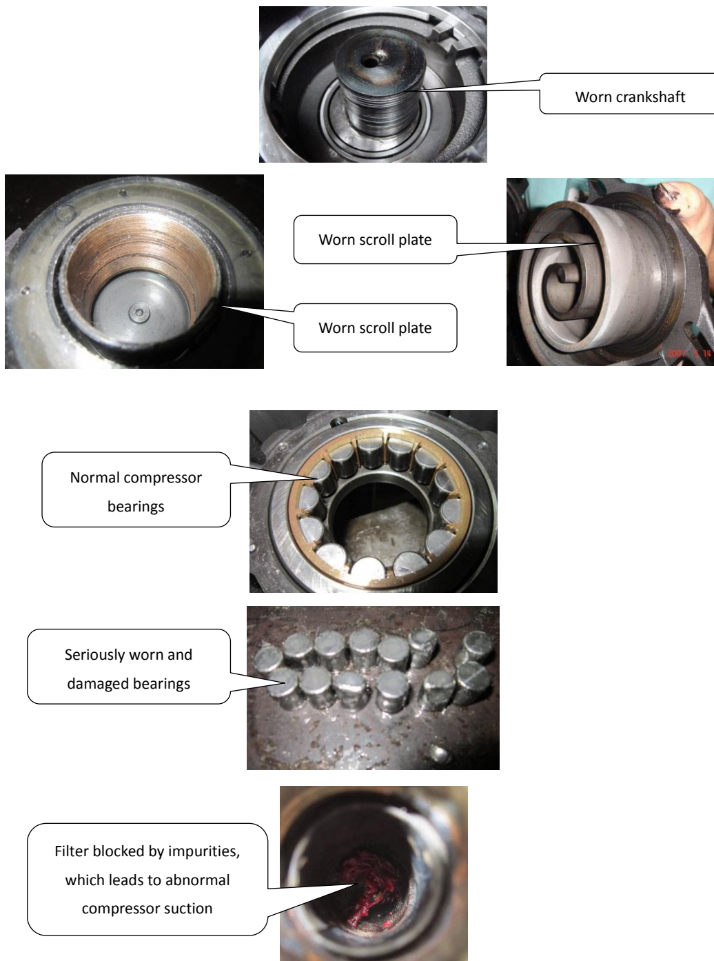
Figure 6-2.11: Effects of spoiled compressor oil
